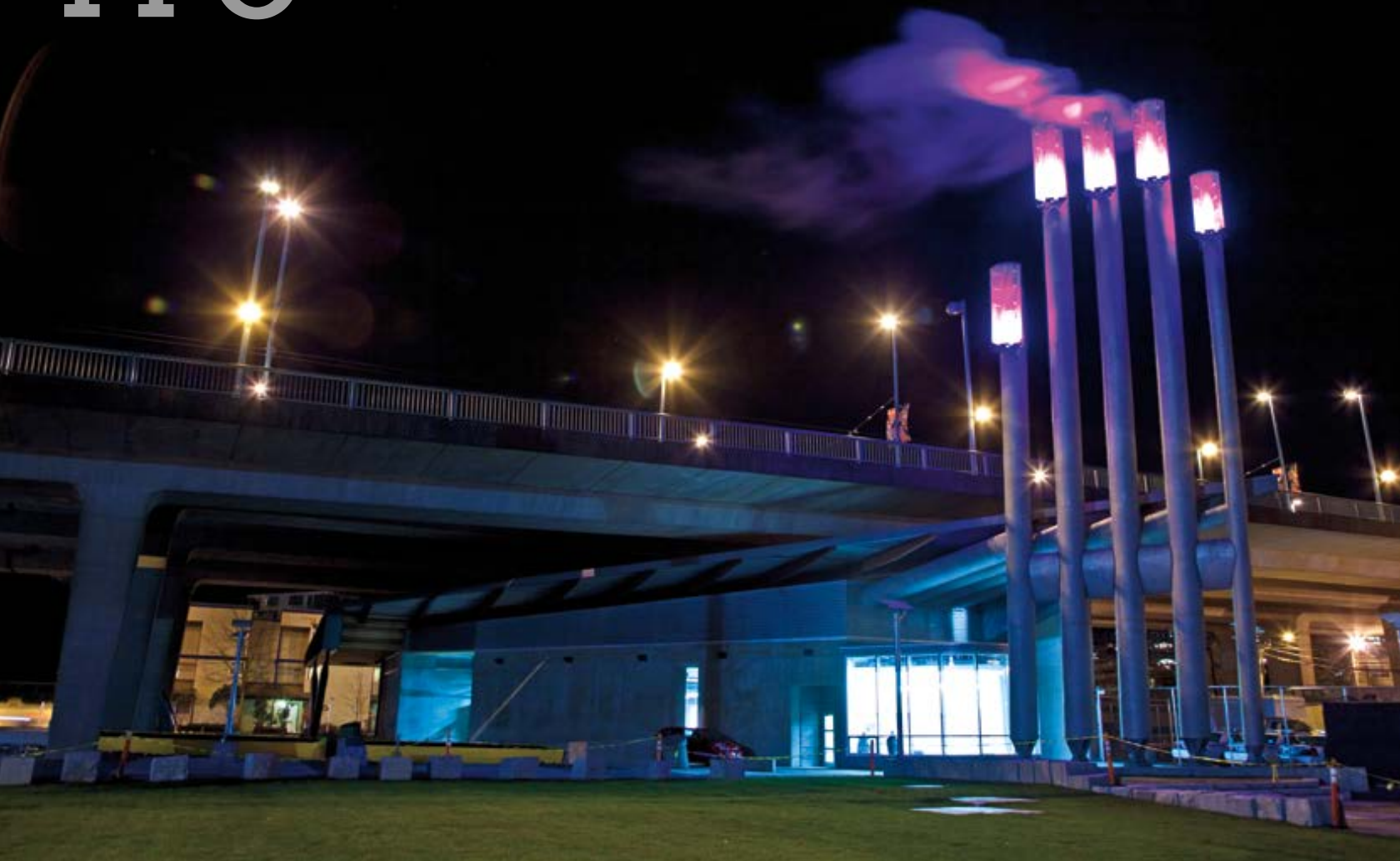
These five exhaust stacks of a plant in Vancouver, BC, that generates energy from sewage are topped with LED lights that change color to indicate energy demand.
